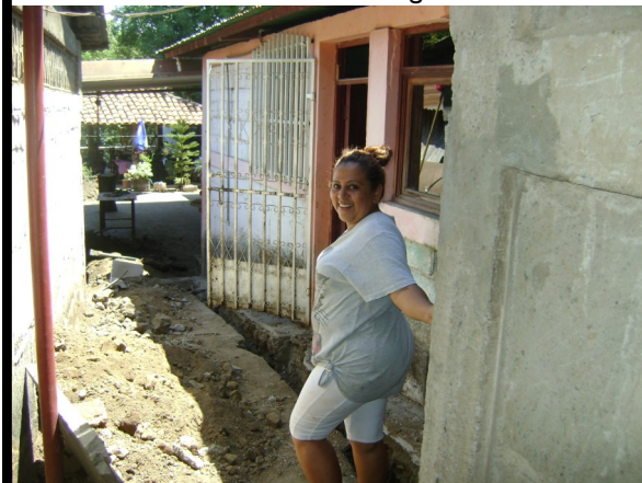
Merla Ruiz Zúñiga in front of the sanitation project
